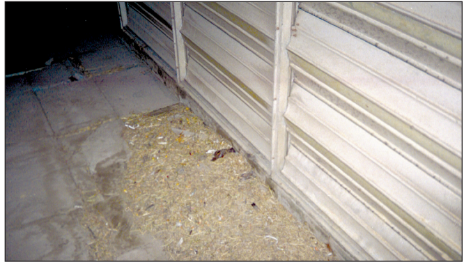
Photo 2: A bird screen failed behind the outdoor air intake louver, allowing organic debris into the air plenum.
